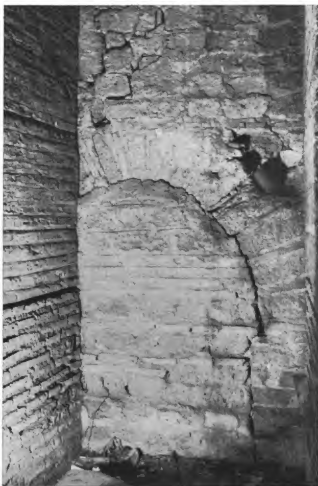
Fig. 227 — S. Maria in Cosmedin. Arched opening in the side wall of the diaconia (Photo: Corbett).
